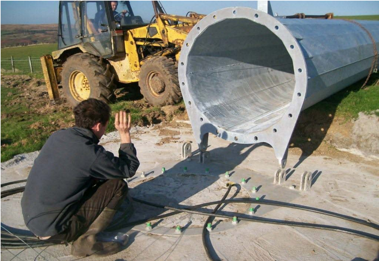
Guiding the Kilmeny turbine into place
