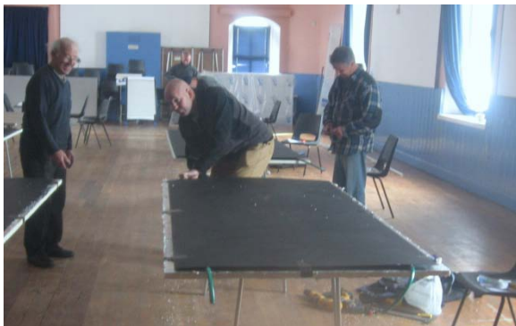
Building solar panels in Bowmore Hall
