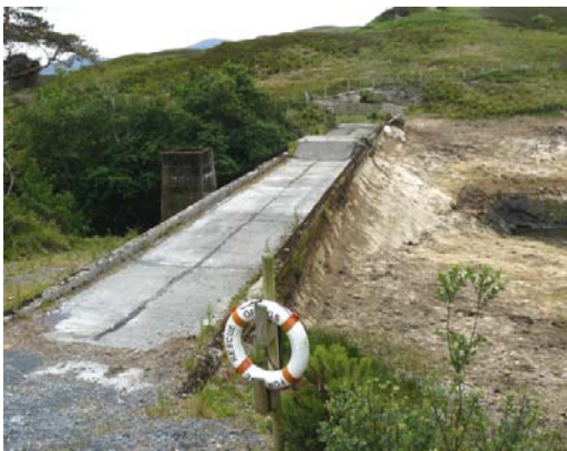
Loch Allan dam drained for inspection
