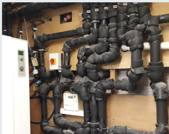
The seven boreholes feed into a 50Kw Nibe heat pump
